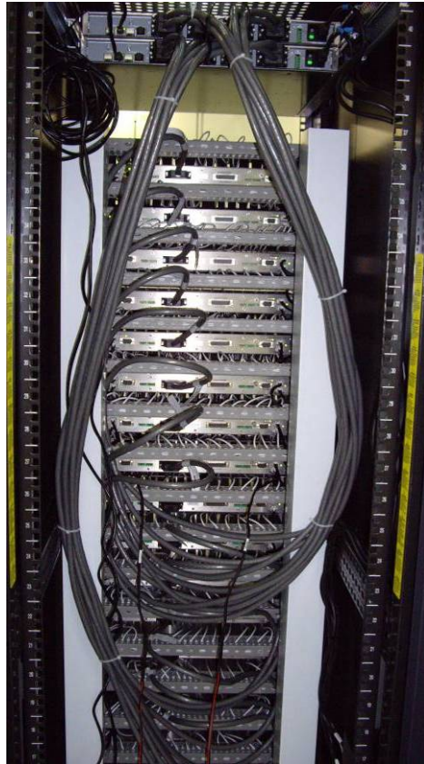
Figure 7: Buffer to Gateway connections – rear view
